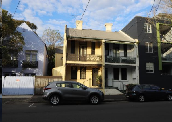
Figure 11: Terrace houses western elevation (Artefact, 2021)
