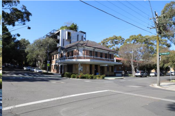
Figure 7: Duke of Wellington north-west elevations (Artefact, 2021)
