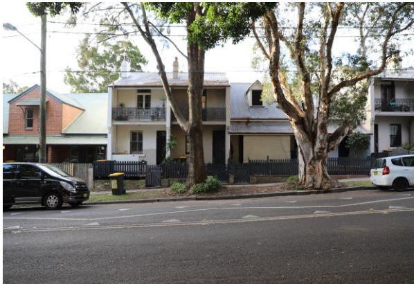
Figure 18: Waterloo HCA terrace houses on Wellington St (Artefact,2021)
