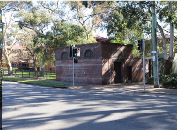
Figure 9: Electricity substation South-eastern elevation (Artefact, 2021)
