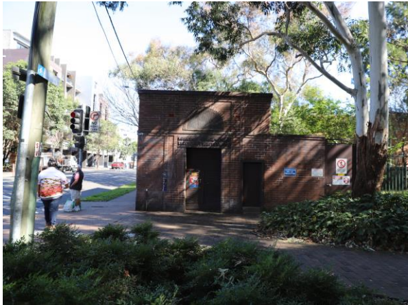
Figure 8: Electricity substation eastern elevation (Artefact, 2021)
